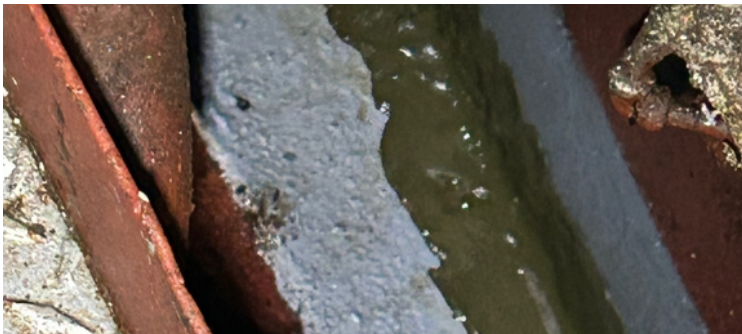
Above: the seam of the transverse bulkhead and hull plating after the application of rust inhibitor and marine epoxy in the aft fire room.
